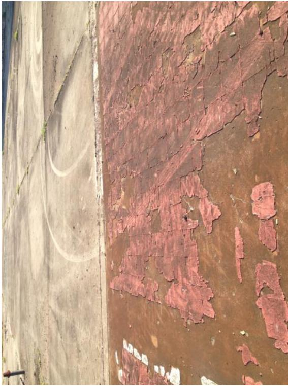
Suspect asbestos-containing tile remnants on foundation
