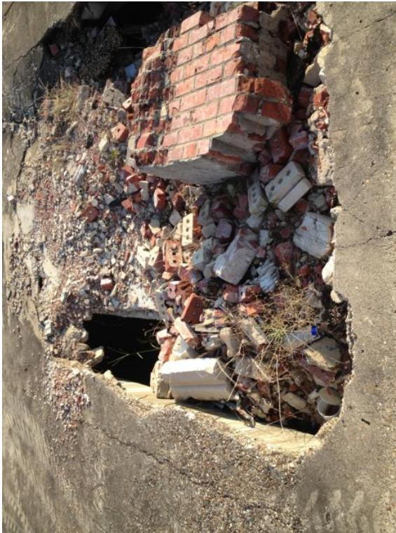
Debris infill of structural failure of above-grade foundation
