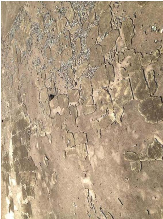
Suspect asbestos-containing tile remnants on foundation
